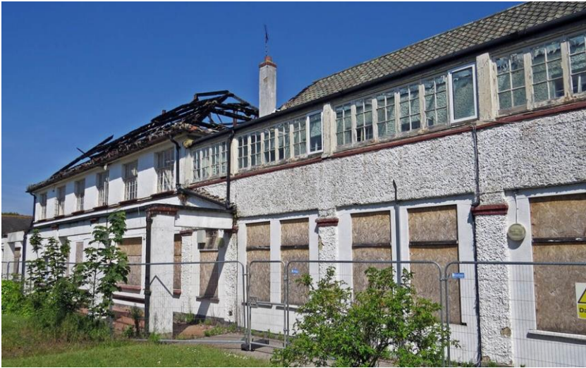
The Old Hospital damaged by fire in 2018
